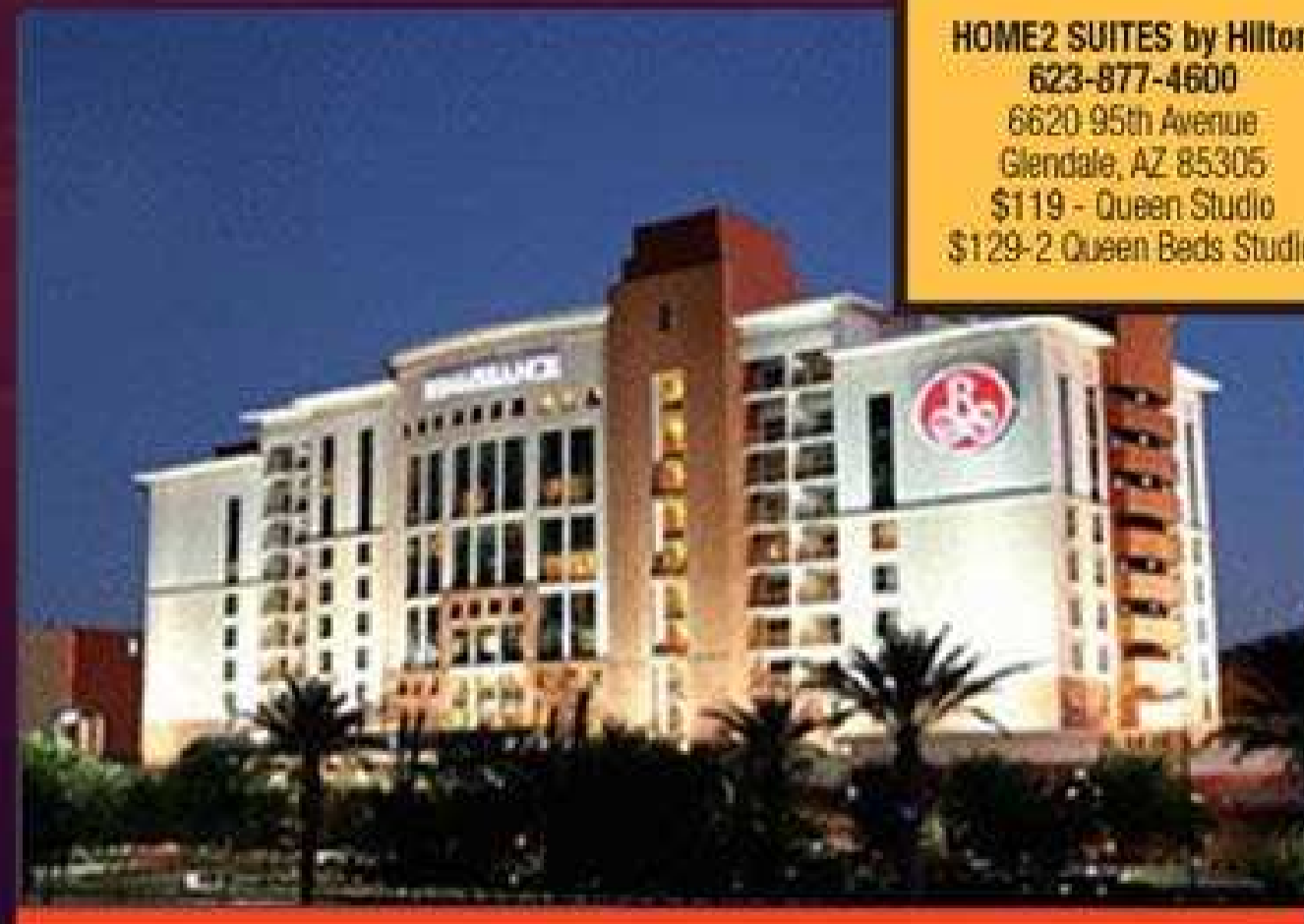
HOST SITE THE RENAISSANCE HOTEL GLENDALE GLENDALE, ARIZONA
